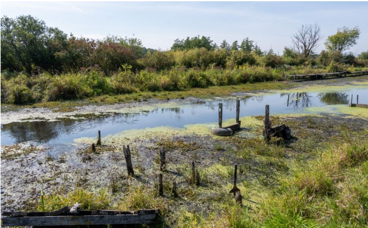
Picture 11: Channelized and widened portion of the stream near the inlet. The former marina areas are full of decomposing, wooden docks and form exposed mud flats during low water. September 16, 2025.
